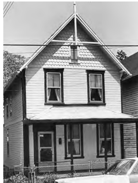
This two-story frame house at 1518 W Street illustrates the quintessential cottage-style dwelling of Anacostia. Its front gable roof and full-width porch feature Eastlake detailing, including fishscale shingles in the gable and a ridge pole.
