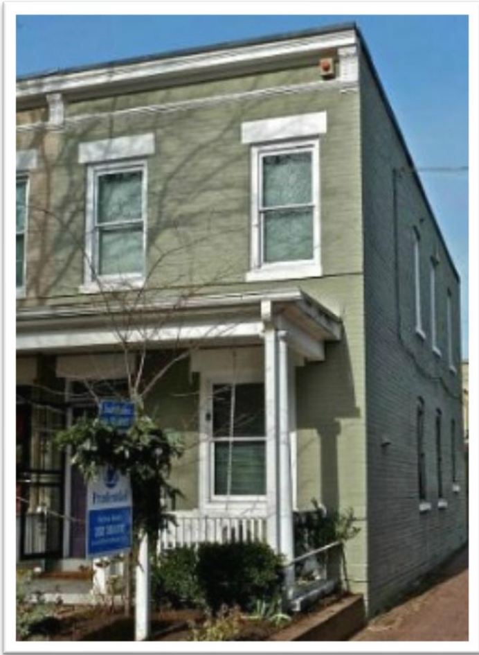
Georgetown (left) and Capitol Hill (right) Federal row houses
