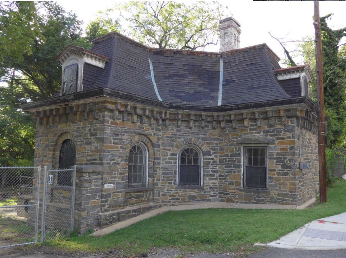
Gatehouse to Corcoran Estate
