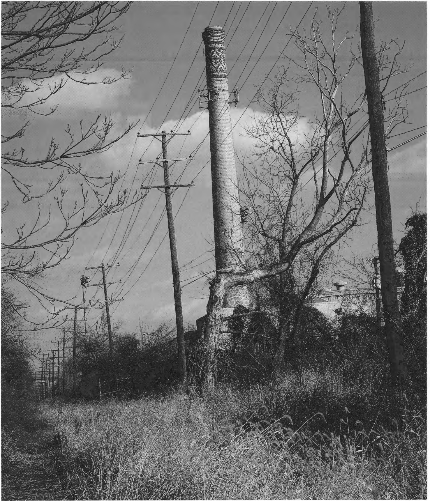
Image 5: Anderson Tire Company, adjacent railroad right-of-way, looking southeast, with rails visible at lower right.
