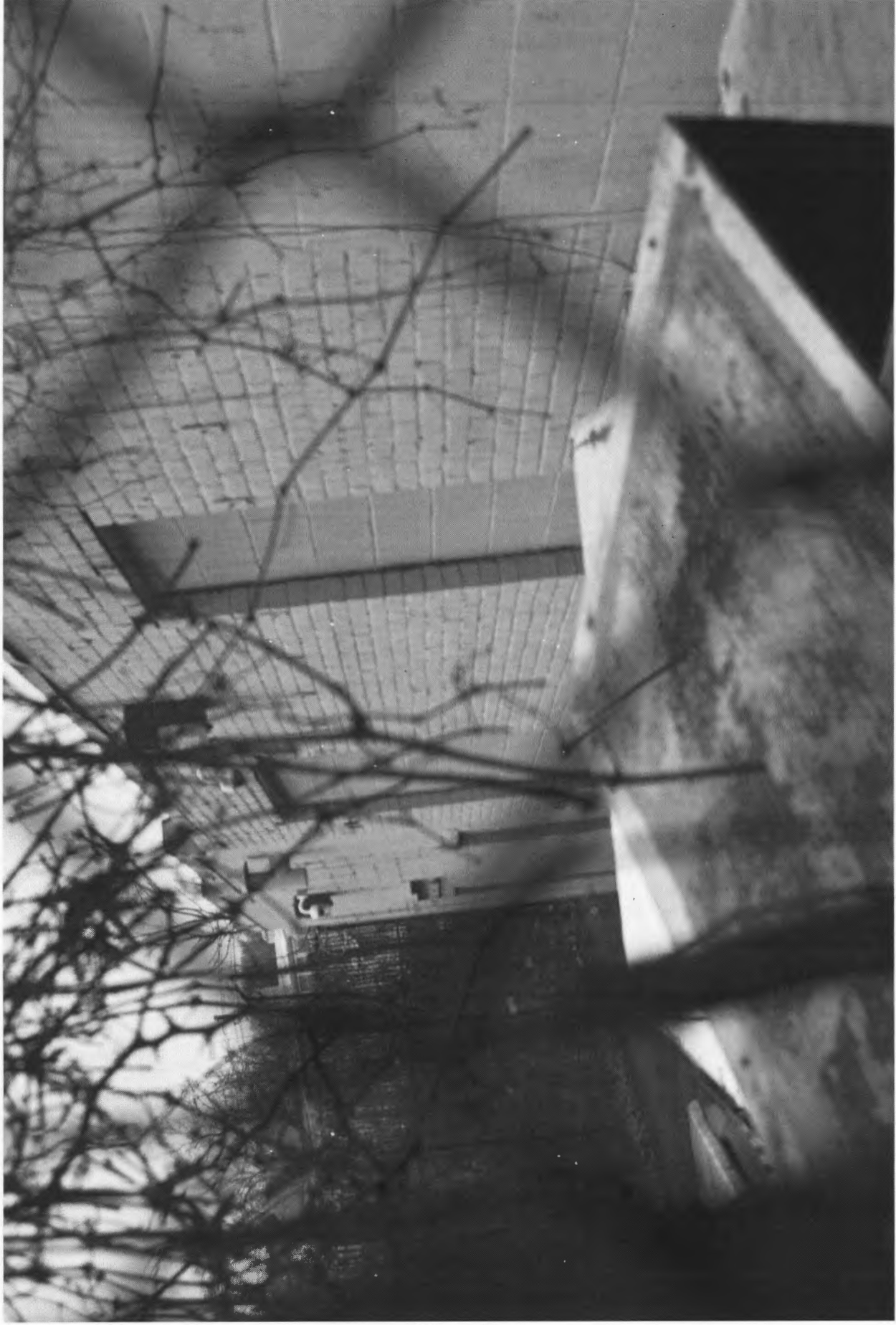
Image 7: Anderson Tire, factory building, east facade.
