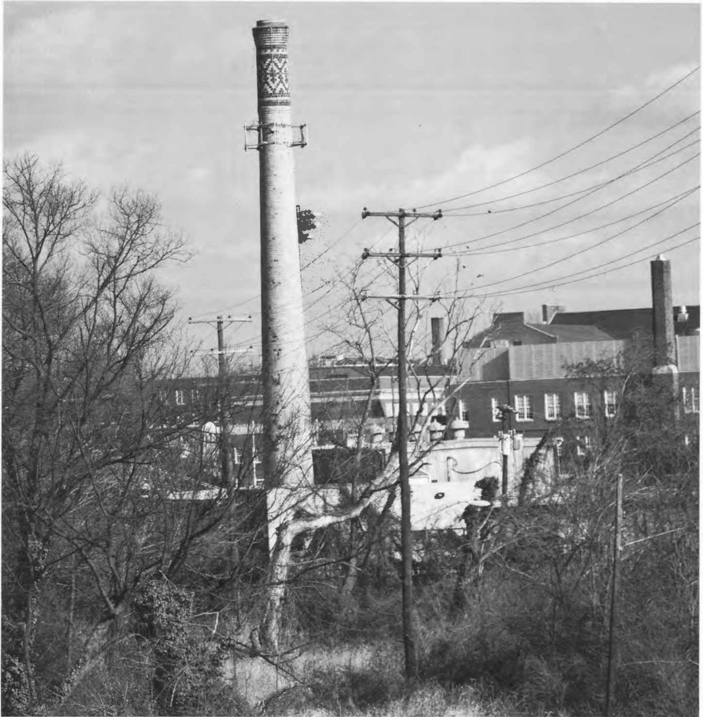
Image 6: Anderson Tire Company, west facade, from bridge above I-295.
