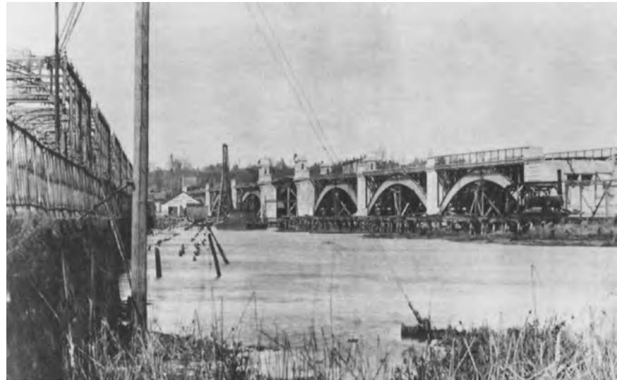
*In 1874, after many years of wooden replacement bridges crossing the Anacostia at the Navy Yard, Congress authorized the construction of a wrought iron truss bridge (at left in photo). As the 1874-75 bridge became inadequate for motor and rail traffic, a new steel arch bridge, shown under construction in this 1908 photograph, was built to replace it. The present, twin-span Eleventh Street Bridge replaced these earlier bridges in 1965-70*
