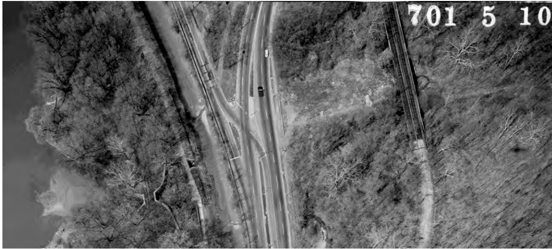
Figure 1.3: Aerial Photograph of the Foundry Branch Bridge circa 1963 (DDOT Archives)
