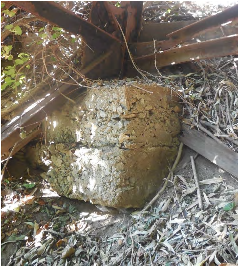
Figure 14: Undercut Footing
