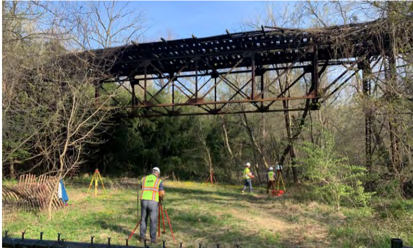
Figure 3.1: Survey Team Performing 3D Scan of the Bridge
