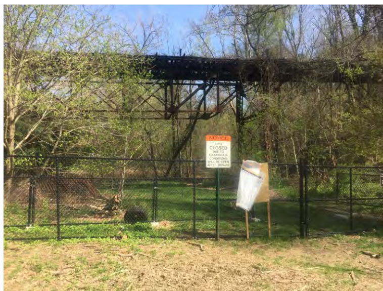
Figure 2.2: Fence and Warning Sign
