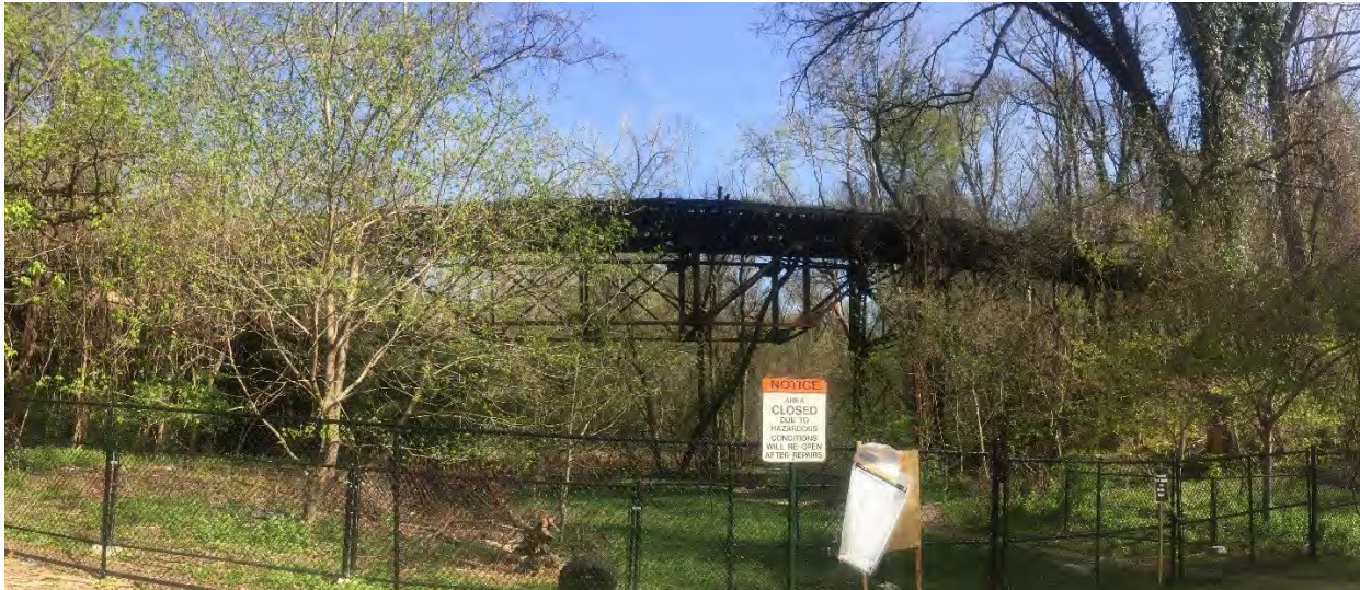
Figure 3: Bridge Elevation Photograph
