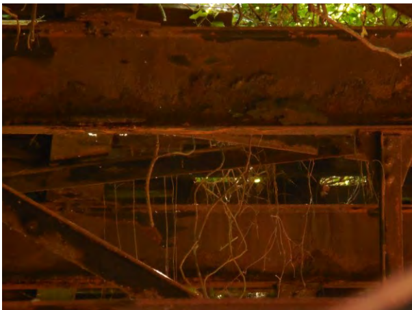
Figure 5.9: Corrosion to 15-inch Deep Cross Girder
