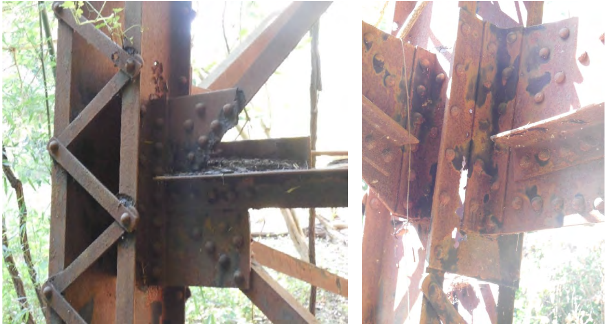
Figure 5.7: Column Connection to Bracing Members
