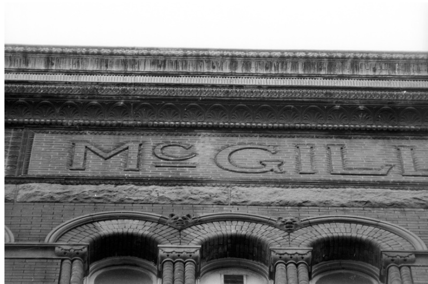
The McGill Building's cornice and intricate brick and stone masonry in 1973, the year that it was demolished. Photo courtesy of the DC Preservation League.
