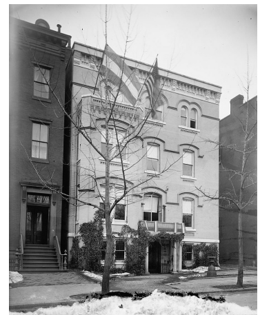
Figure 3-9. National Woman's Party Headquarters at 14 Jackson Place ca. 1918-1920, demolished (Library of Congress).
