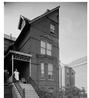
Figure 4-5. Mary Church Terrell House at 326 T Street NW in 1933 (Library of Congress).
