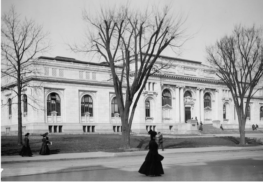
Figure 2-8. DC Central Public Library, where some suffrage and anti-suffrage meetings were held (Library of Congress).
