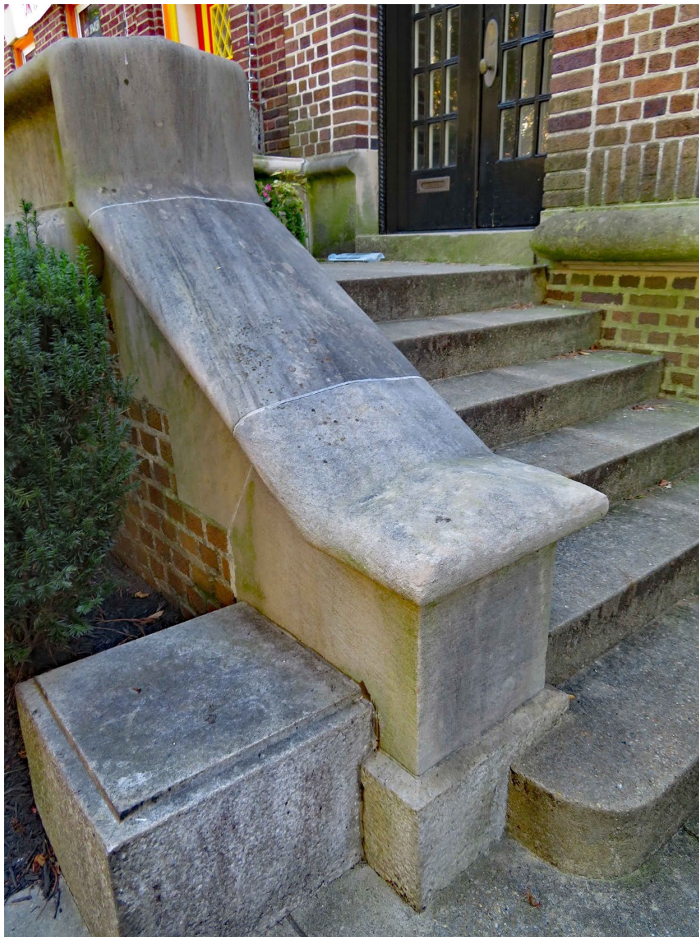
Photo A3: Front staircase and entry porch (J. DeFerrari).
