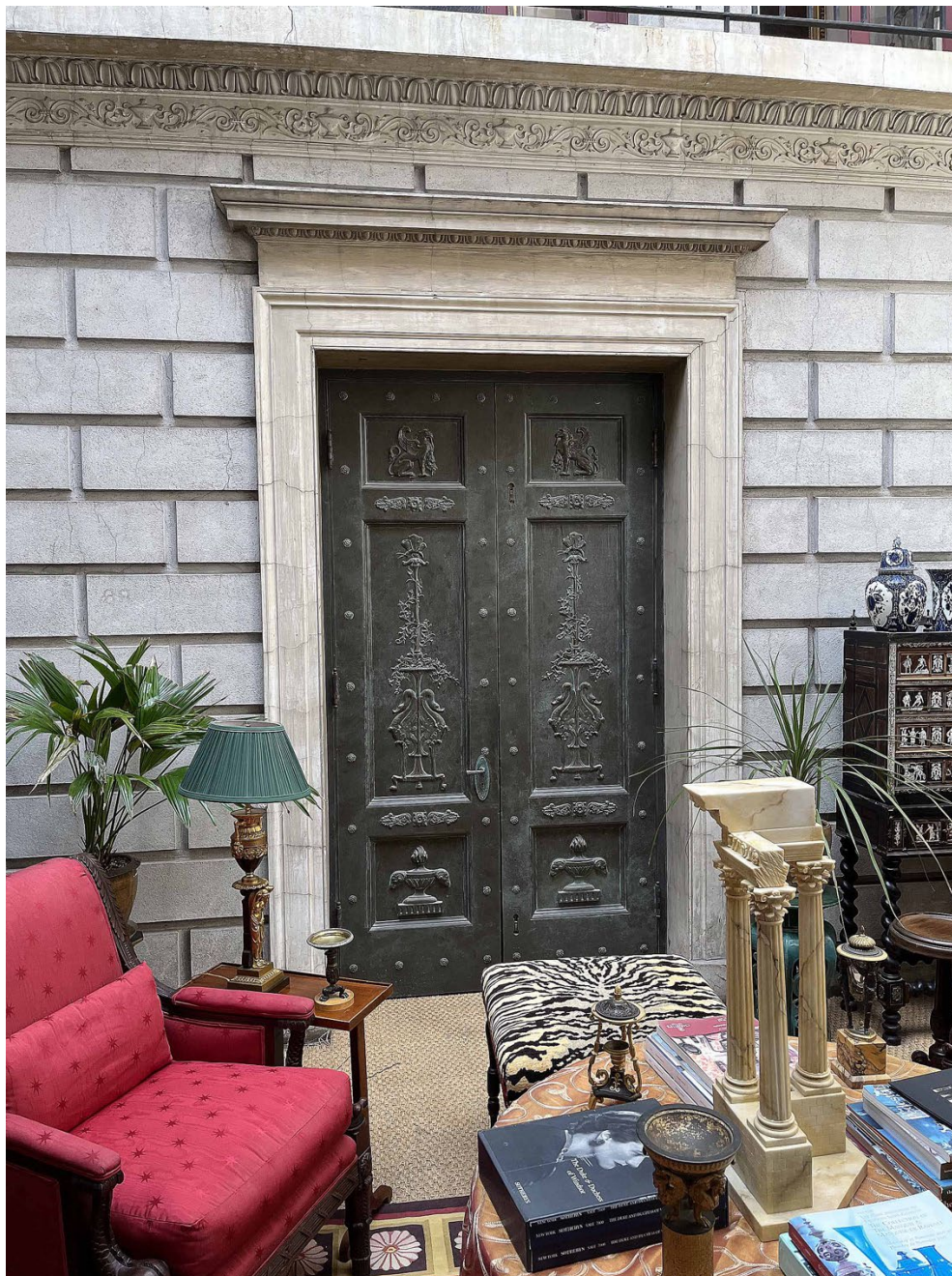
Photo E5: Atrium west wall with non-original door (J. DeFerrari).
