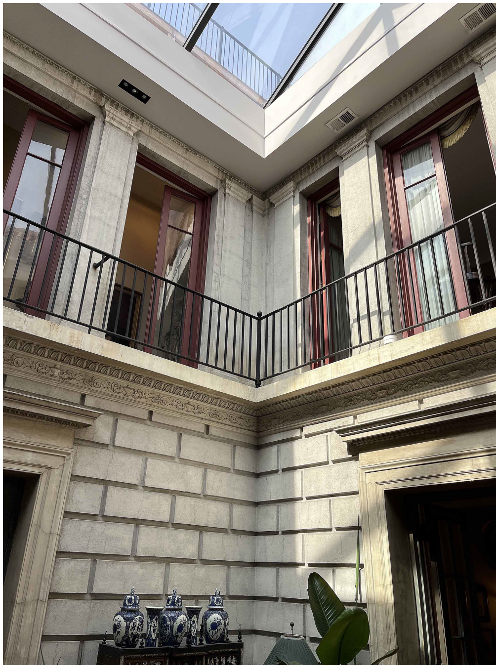
Photo E4: Atrium northwest corner (J. DeFerrari).
