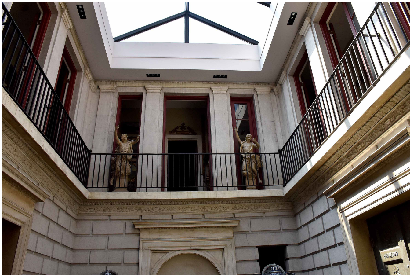
Photo E6: Atrium second story balcony south wall (D.P. Sefton).
