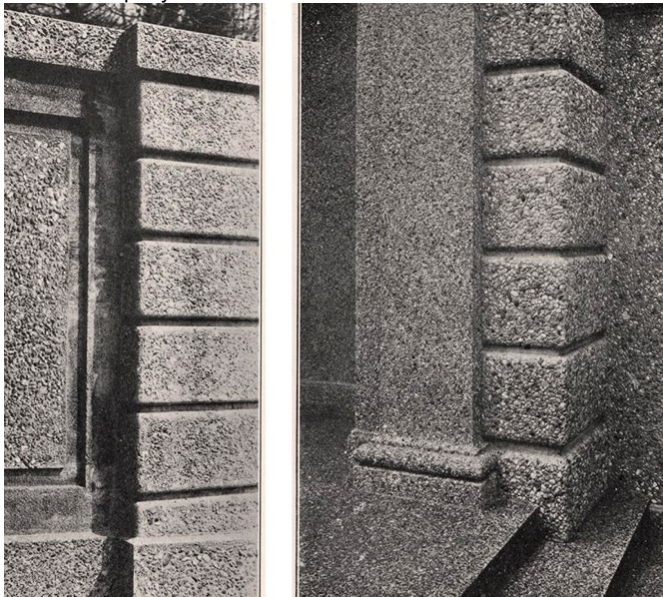
Figure 3: Patterned Concrete Walls at Meridian Hill Park. Source: Horace W. Peaslee. "Notes On the Concrete Work of Meridian Hill Park, Washington," Landscape Architecture Magazine , Oct. 1930, Vol. 21, No. 1, p. 34.
