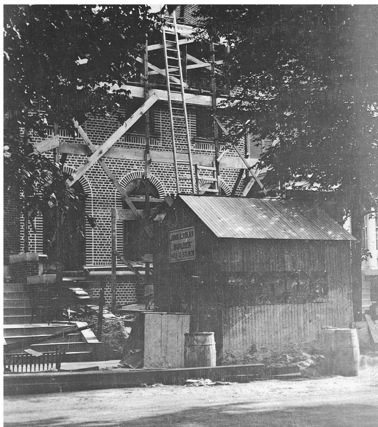
Figure 2: 1710 Lamont Street NW under construction, c. 1911 (David Alfuth collection).
