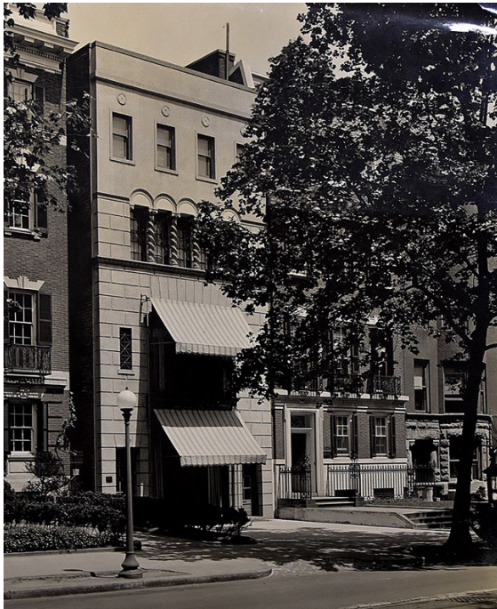
Figure 4: Façade at 3300 Connecticut Avenue Showing Concrete Detail, 1923. Source: Frederick W. Cron - John Joseph Earley collection, Georgetown University Booth Family Center for Special Collections.
