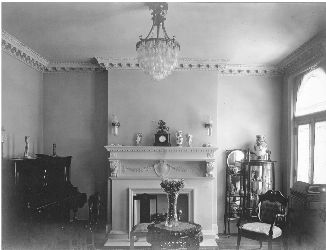
Photo C1: Historical photo of Parlor mantle and fireplace, west wall (David Alfuth collection).
