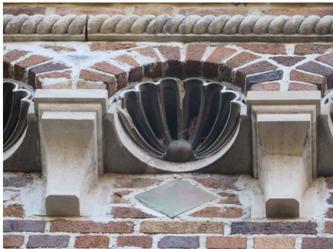
Figure 1: Detail of decorative concrete shell with ventilation slats (J. DeFerrari).
