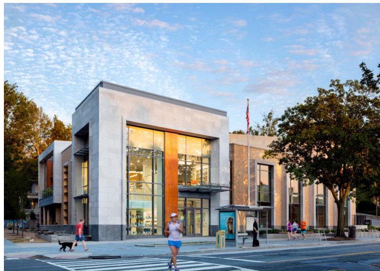
Exterior of the Cleveland Park Library. Photo courtesy of the DC Public Library.
