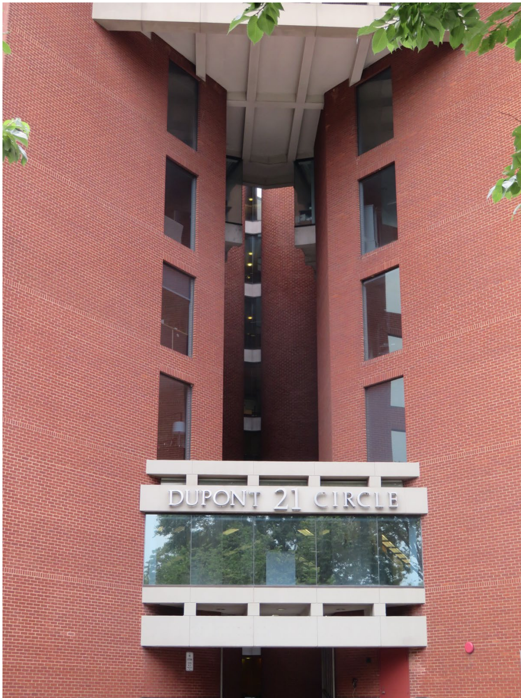
Photo 5: Euram Building (21 Dupont Circle), detail of façade (north elevation) (J. DeFerrari).
