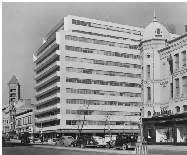
Figure 6: The Longfellow Building as it originally appeared in the 1940s. Modernist ribbon windows like these also appear on the Euram Building. (Source: Library of Congress).
