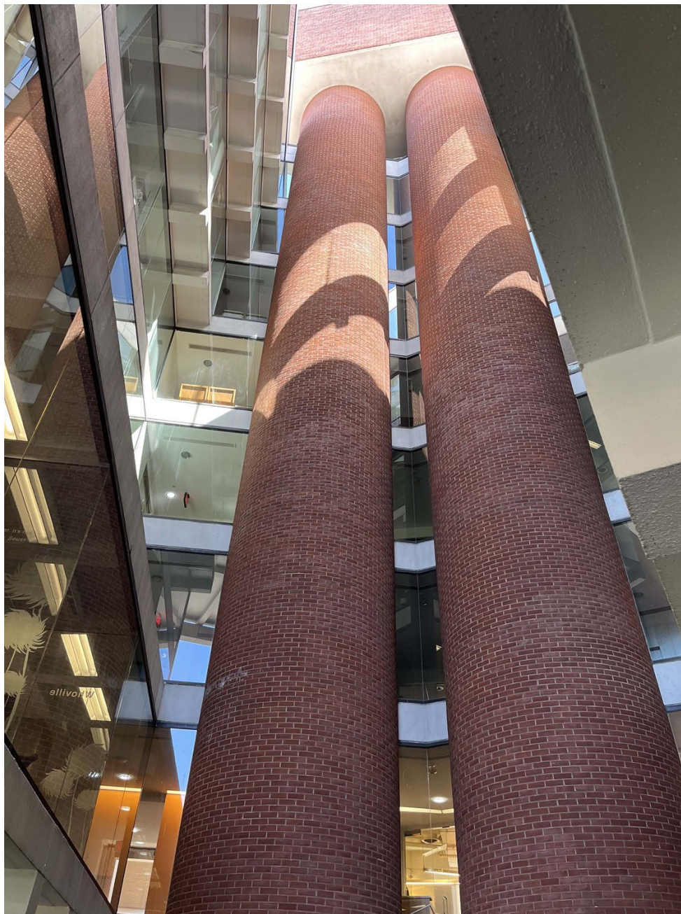
Photo 12: Alternate view of cylindrical elevator towers and upper floors from the interior courtyard, facing south. (J. DeFerrari).
