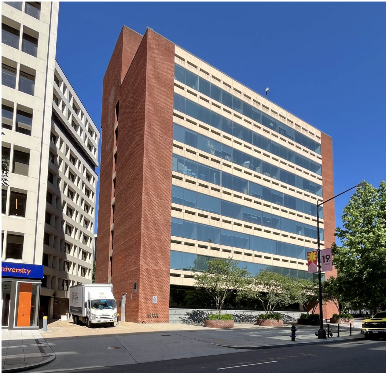
Photo 7: Euram Building (21 Dupont Circle), east elevation and partial view of south elevation facing alley (J. DeFerrari).
