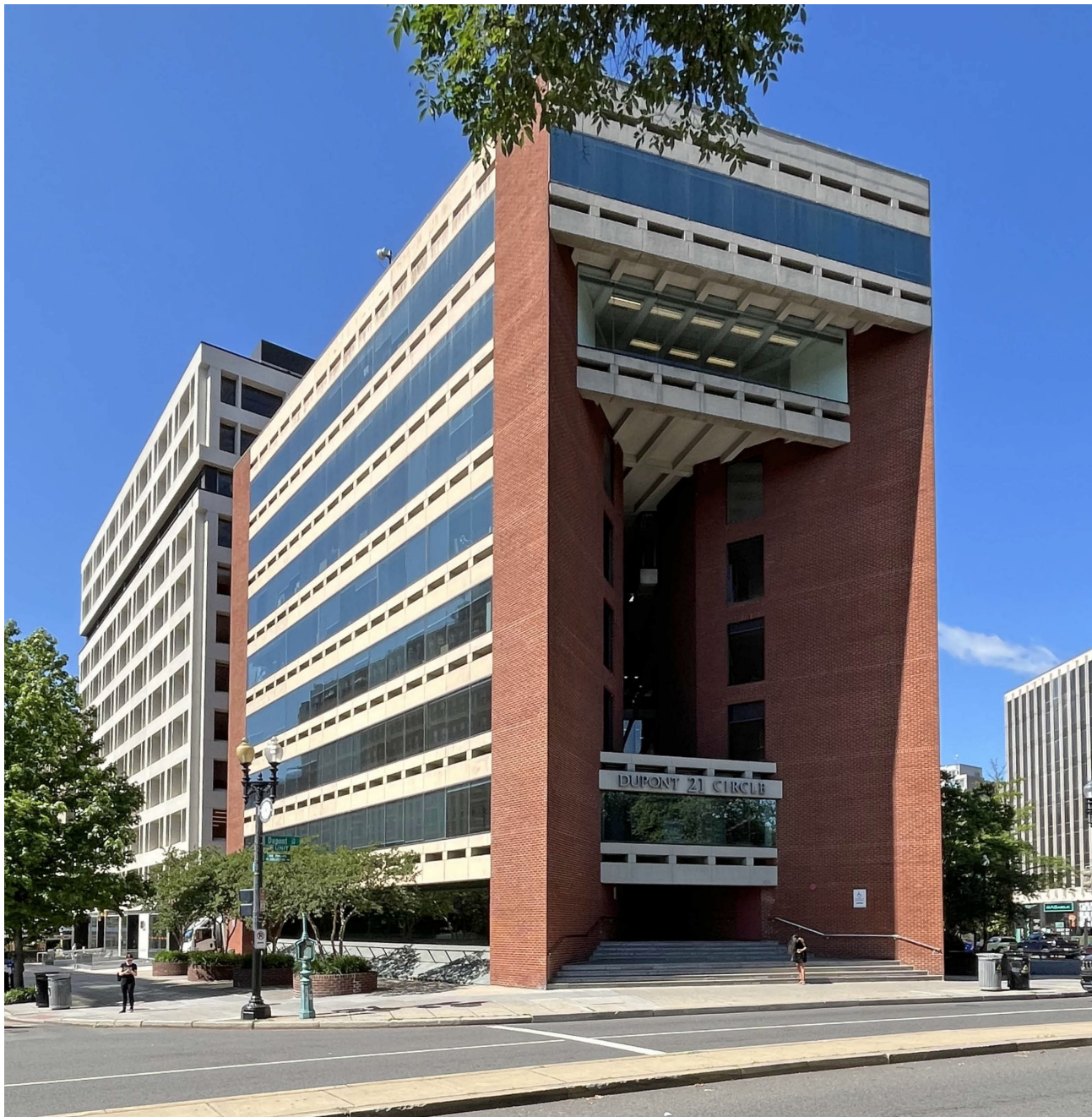
Photo 3: Euram Building (21 Dupont Circle), façade (north elevation) and east elevation, seen from Dupont Circle (J. DeFerrari).
