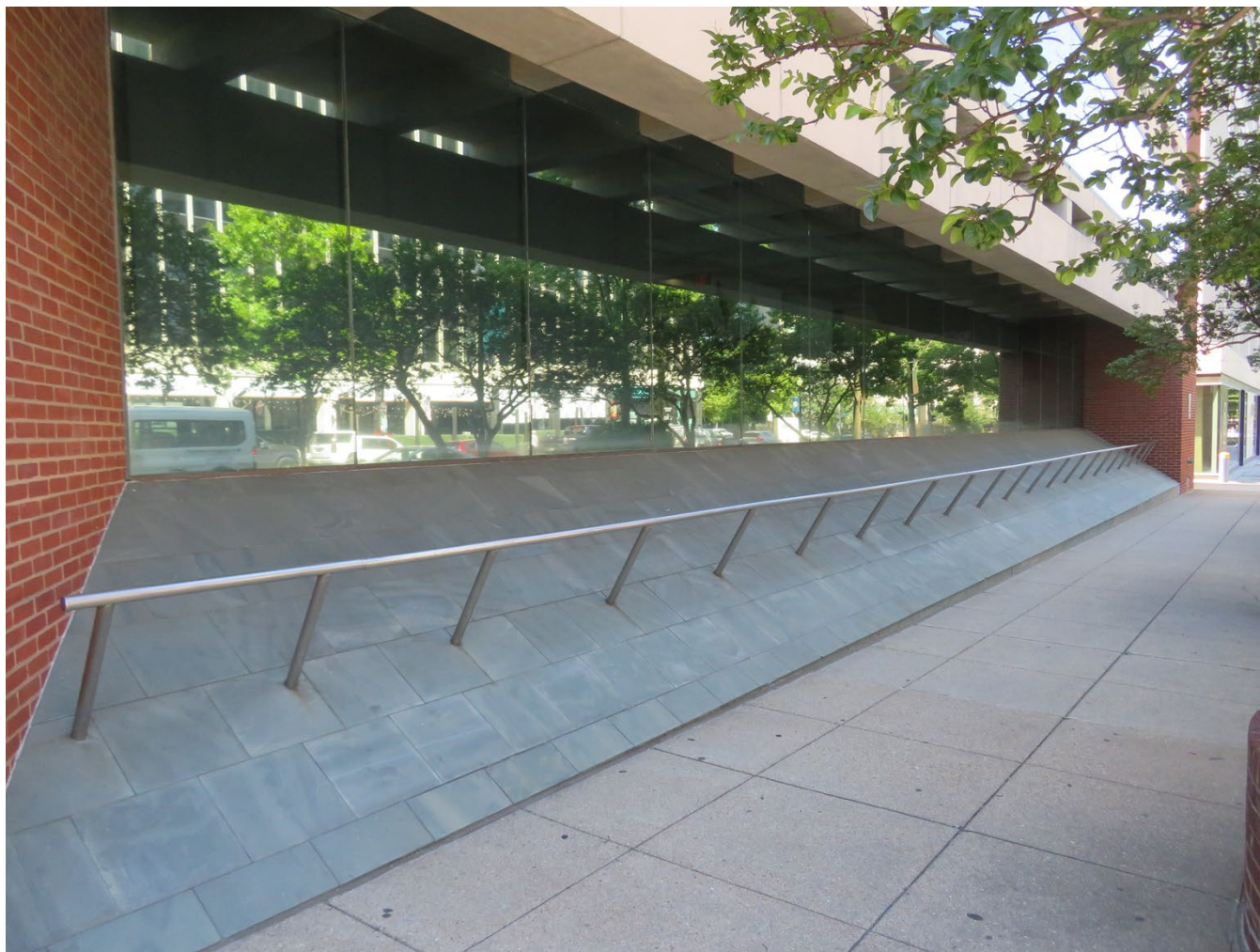
Photo 8: Detail of ground level, west elevation (J. DeFerrari).
