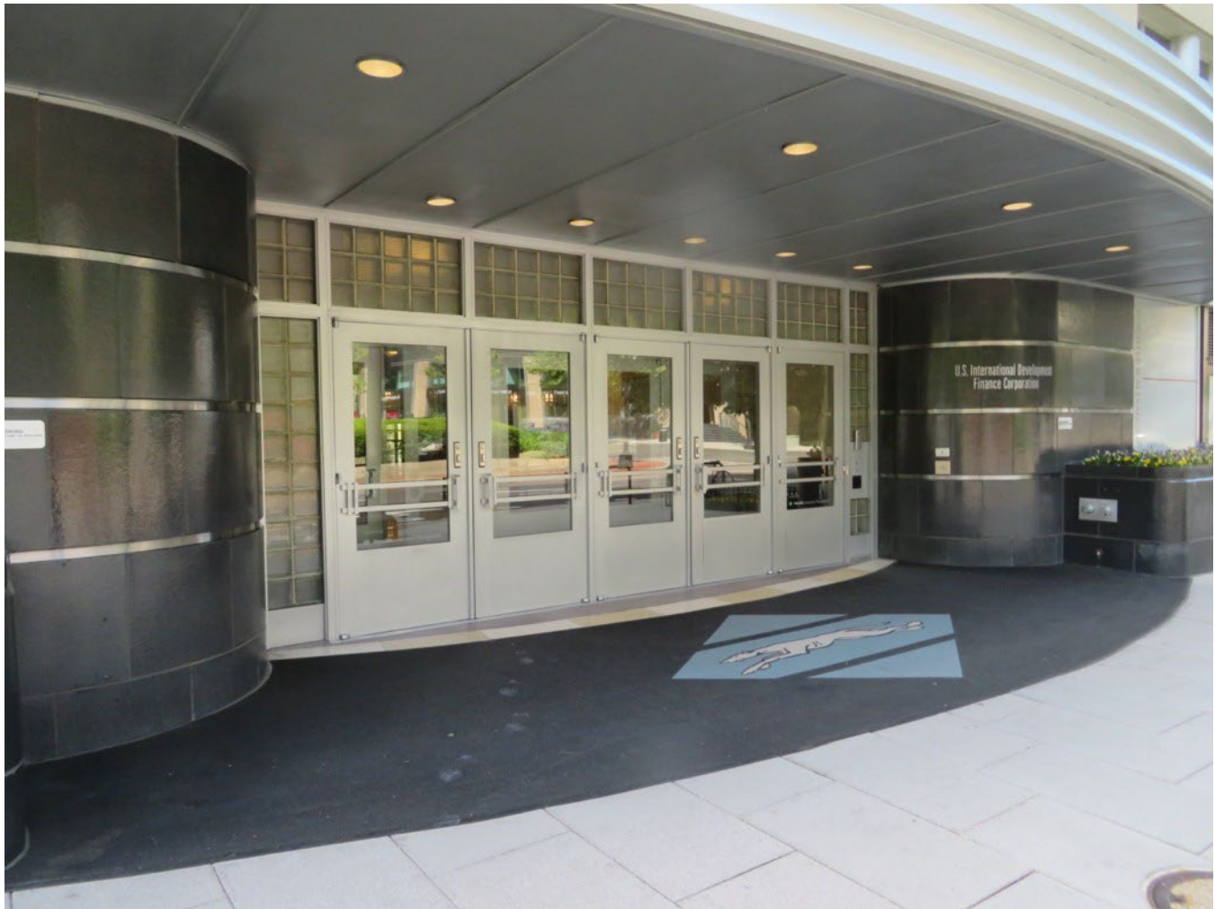
Photo 10: Detail of main entrance, 4-26-2024. (J DeFerrari).
