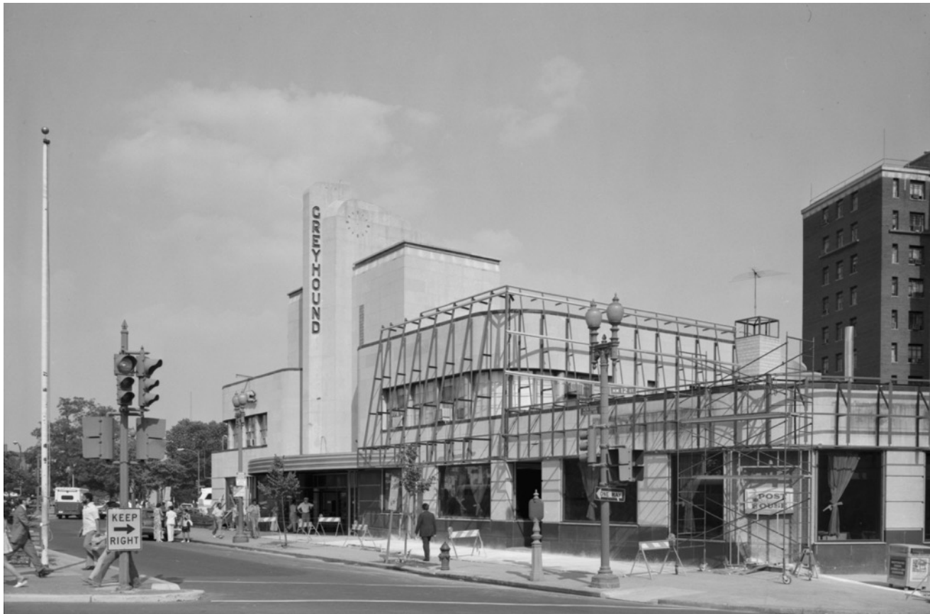
Photo 3: View of the façade of the Greyhound Terminal during modifications, facing southeast, June 1976. (Jack E. Boucher, Historic American Buildings Survey).
