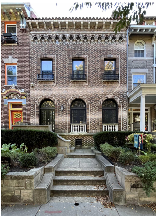
Photo of Front Elevation of John Joseph Earley House, 1710 Lamont Street NW. Photo by John DeFerrari.
