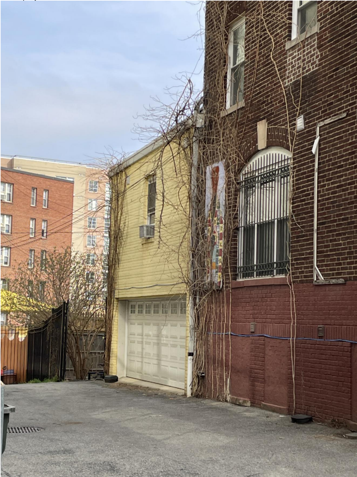
Photo 5: DC_LAYC_0005.tif: View facing southeast of attached garage north elevation
