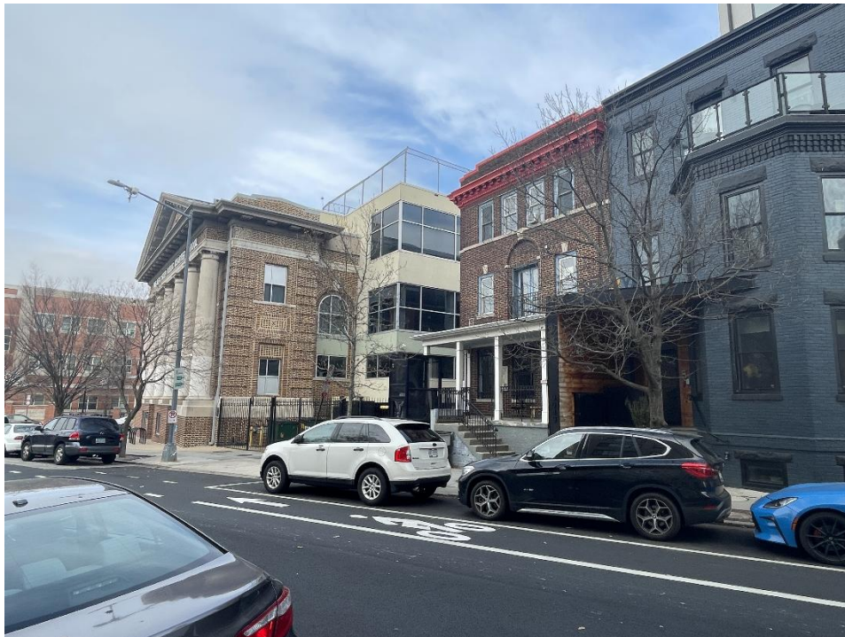
Photo 3: DC_LAYC_0003.tif: View facing northeast of west elevation from 15 th St. NW
