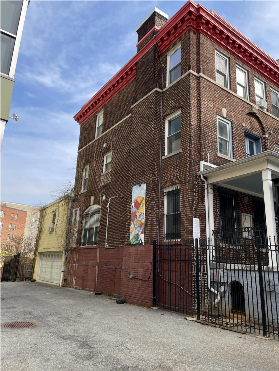
Photo 4: DC_LAYC_0004.tif: View facing southeast of north elevation
