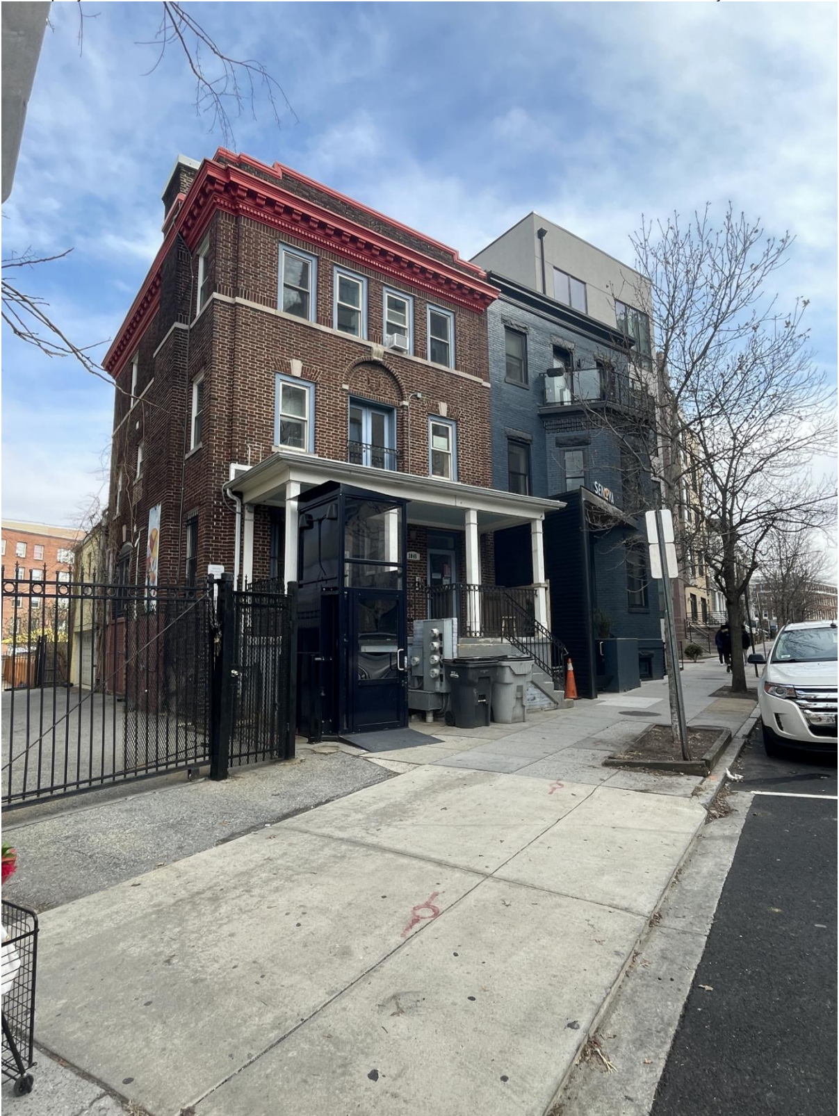
Photo 1: DC_LAYC_0001.tif: View facing southeast of northwest elevation
