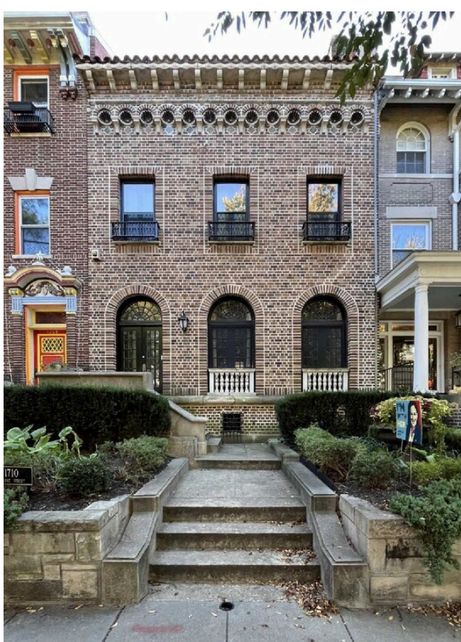
John Joseph Earley House at 1710 Lamont Street, NW; Designated with Interior Spaces in 2025; Photo by John DeFerrari
