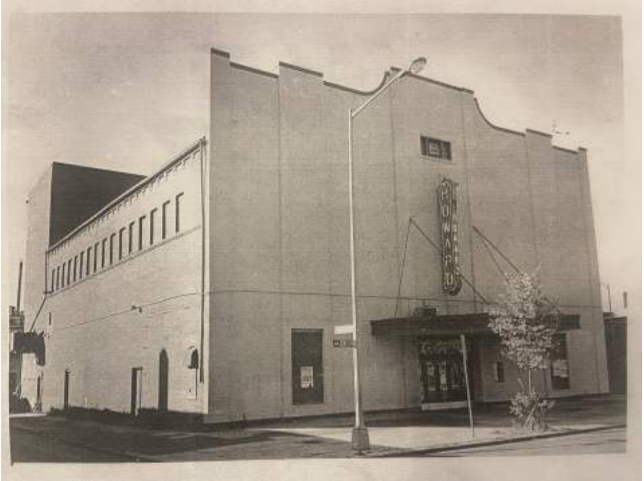
Figure 10. North and east elevations, 1978 (Washingtoniana Division, Martin Luther King Jr. Memorial Library)
