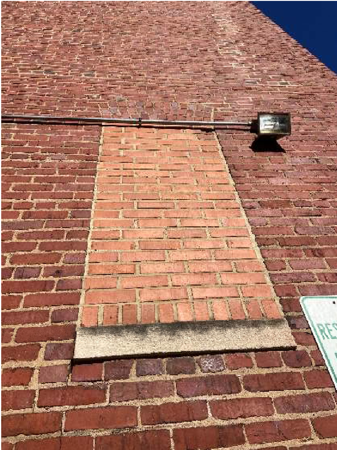
Photo #10 DC_Howard Theatre_0010 South elevation, looking north
