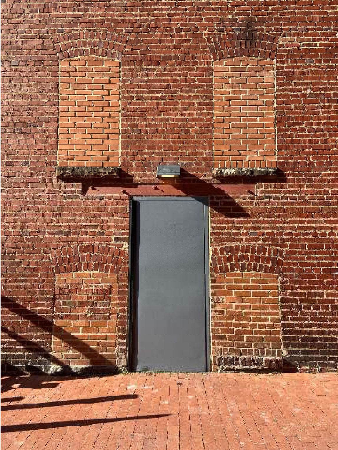
Photo #9 DC_Howard Theatre_0009 East elevation, looking west
