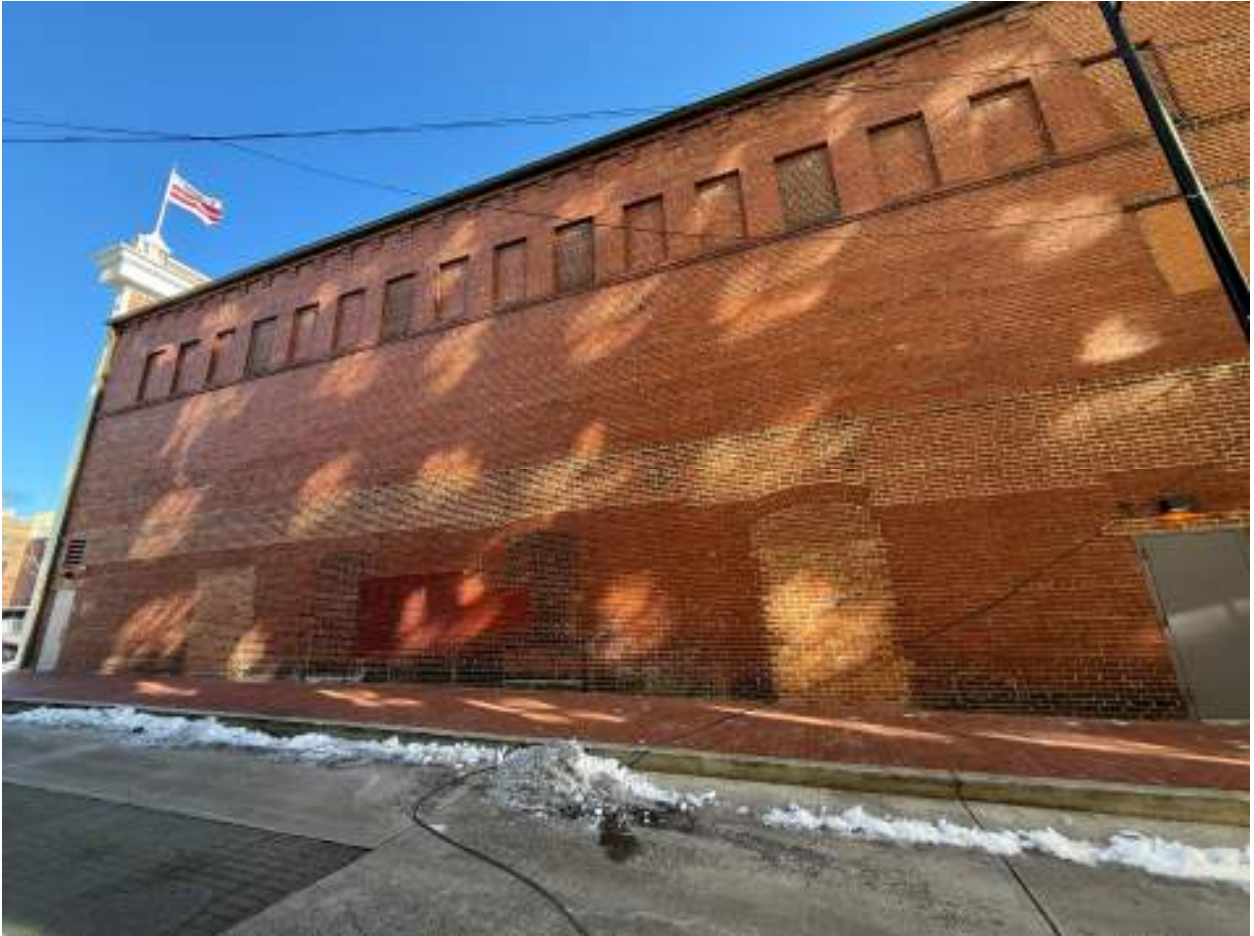
Photo #4 DC_Howard Theatre_0004 West elevation, looking northeast
