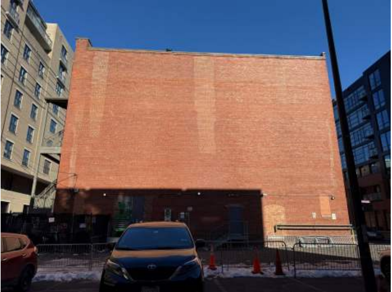
Photo #3 DC_Howard Theatre_0003 South elevation, looking north
