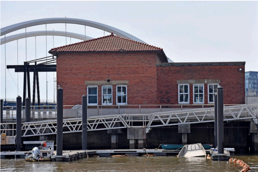
View of the Capitol Power Plant Pump House, which sits above the Anacostia River. Photo by D. Peter Sefton.
